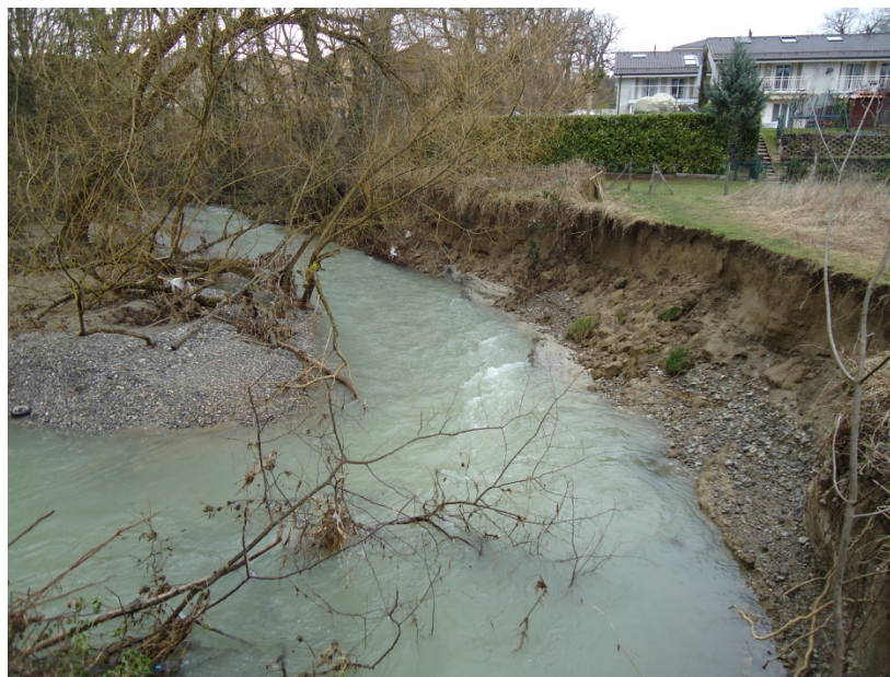
Figure 6 Unstable bank at around 4km of the D/S end (Photo was taken on 4.03.2014)
