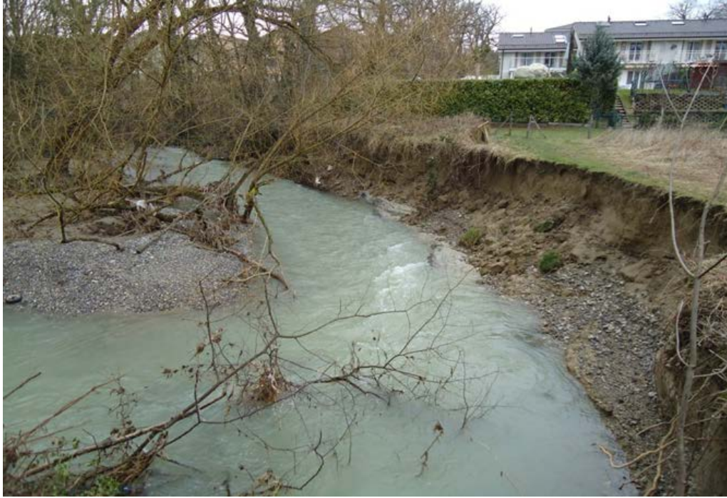
Figure 6 Unstable bank at around 4km of the D/S end (Photo taken on 4.03.2014).
