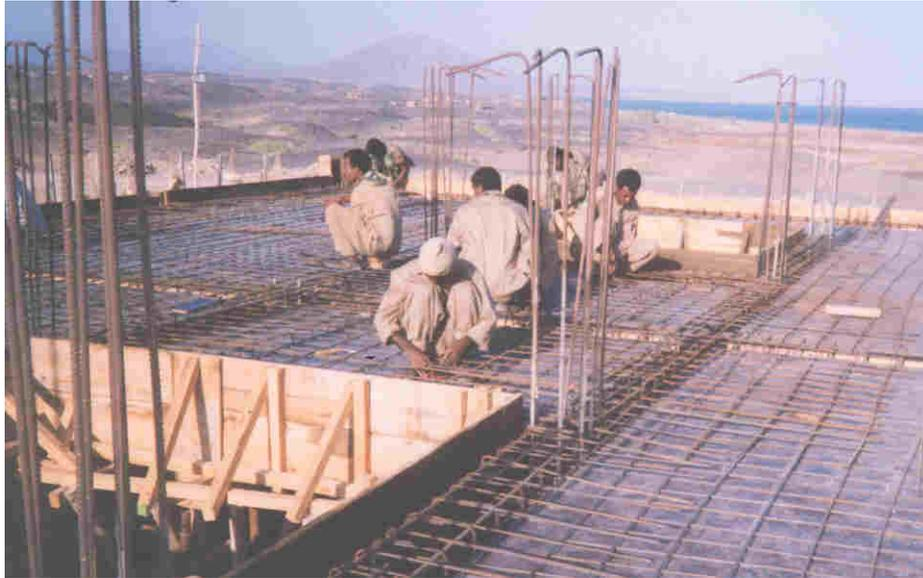
Figure 9 First floor reinforcement placement
