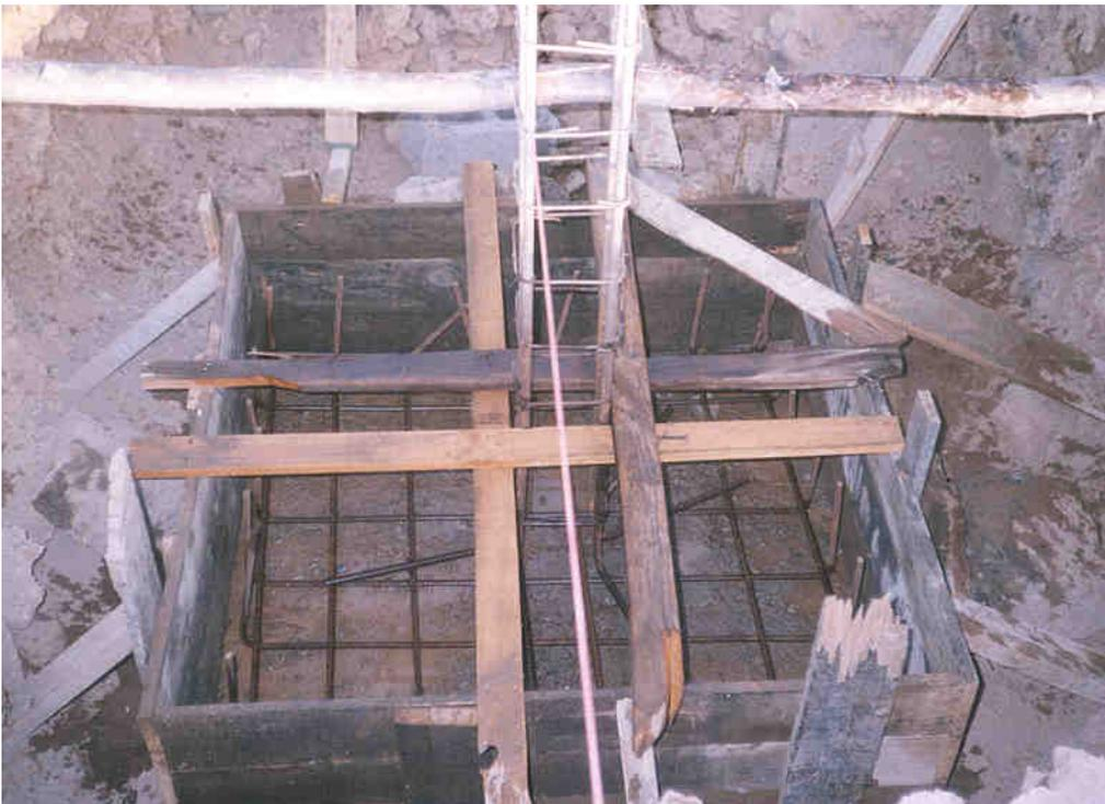
Figure 4 Single spread foot foundation utilized at Assab hospital
