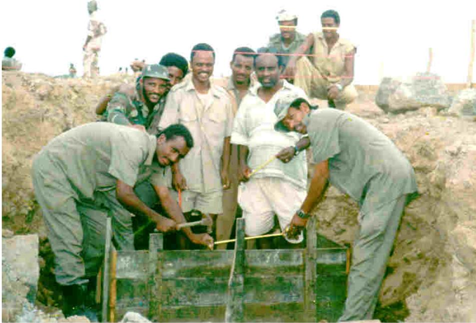
Figure 5 Foundation formwork placement
