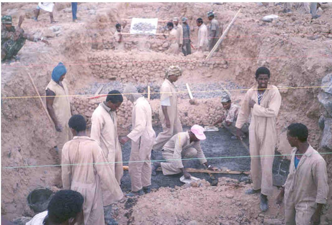
Figure 2 Lean concreting at Assab construction site
