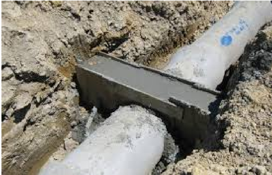
Figure 5 Seepage protection collar
