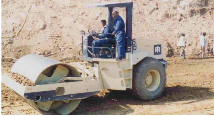
Figure 9 Compaction of Halhal dam
